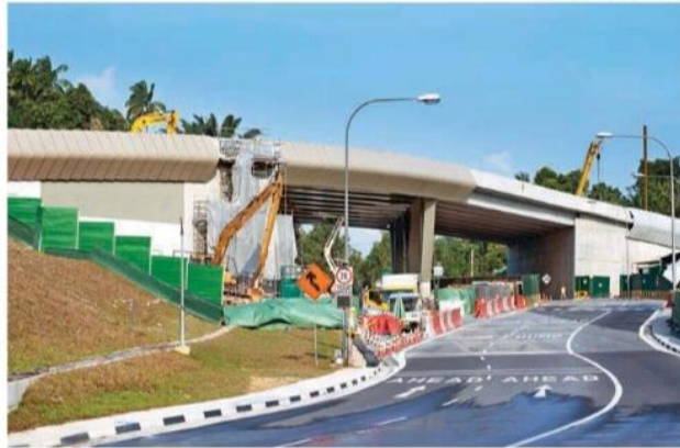
An elevated wildlife crossing being built across Mandai Lake Road
