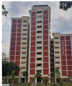
Photo 6: Colour zoning, enlarged block numbers and contrasting colored vertical strips to the public housing estates to help better wayfinding within the neighbourhood.
